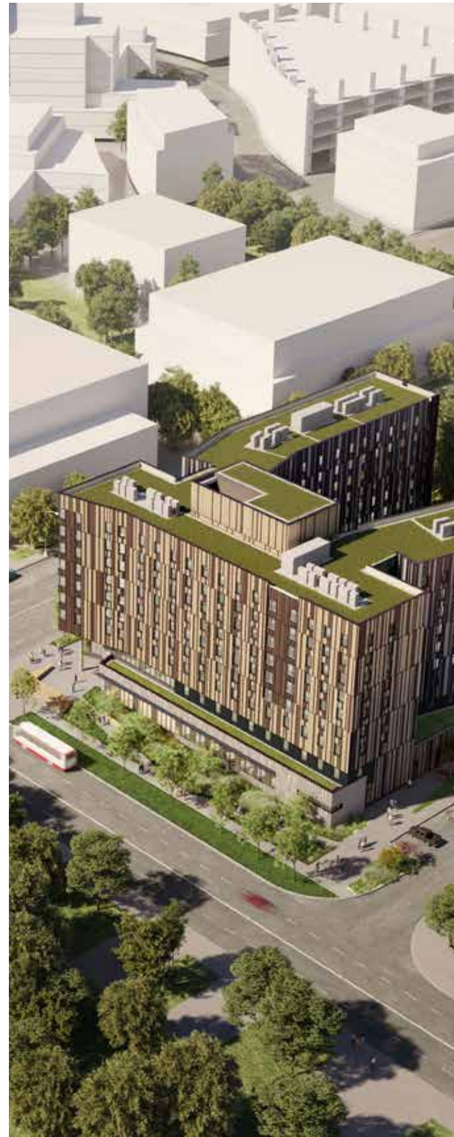
The University of Toronto Scarborough Campus (UTSC), a 750-bed Passive House Student Residence, designed by Arcadis.
