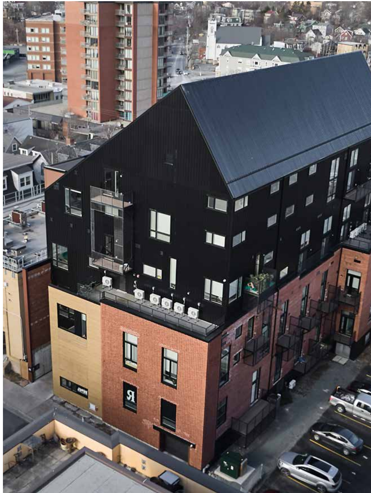
36 Wentworth Street, Dartmouth, Nova Scotia: Once a forgotten telecom storage site, Tel Lofts is now home to 24 of downtown Dartmouth's most unique hard loft units.
