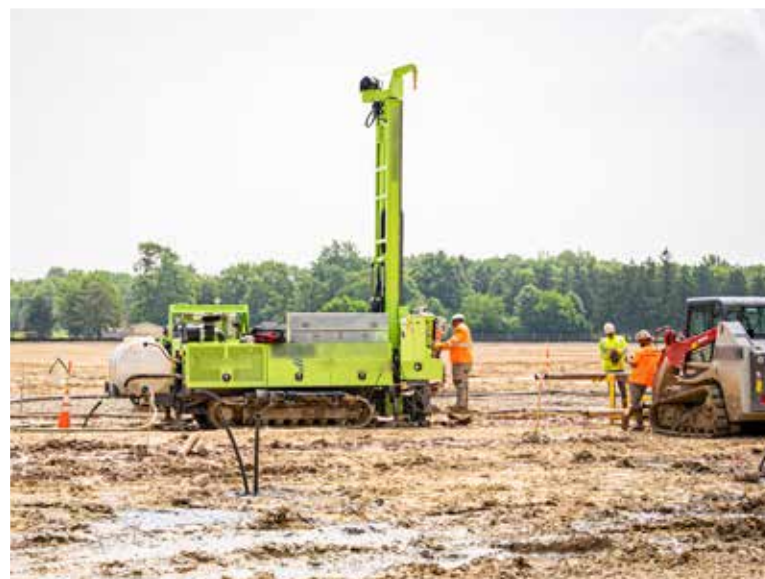
A Subterra geothermal drilling project located in Toronto, Ontario.
